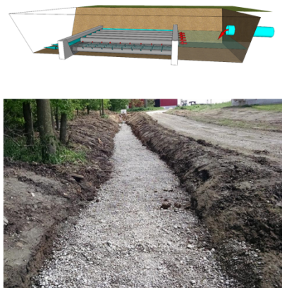
Layout and photo of installed ditch-style P-filter
